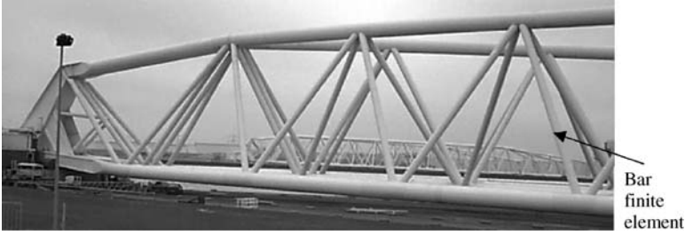
Figure 2.1 A bridge truss.
