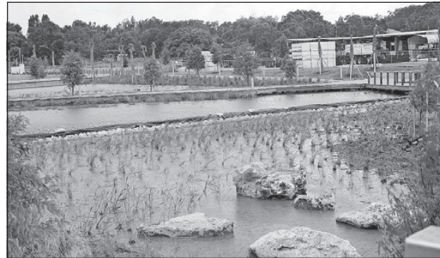
The stream bed at Victory Pointe has been fully planted with aquatic plants and the sandbags that temporarily built up the weir so that workers could set the plants has been removed. [LINDA CHARLTON / CORRESPONDENT]
