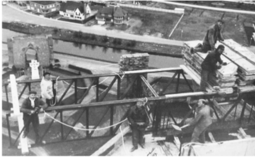
Figure 7. Trusses forming the arms of the cross; prefabricated brick-and-concrete slabs, ca. 1964 (Collection Karel Canfyn).
