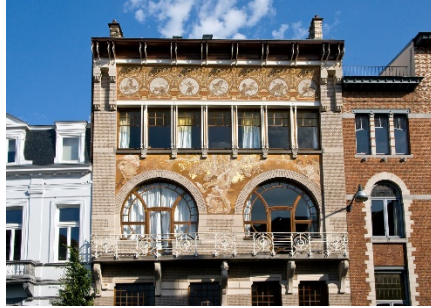
Paul Hankar: Ciamberliani house, rue de Faqz, Brussels, 1897. [recent photograph by ed.]
