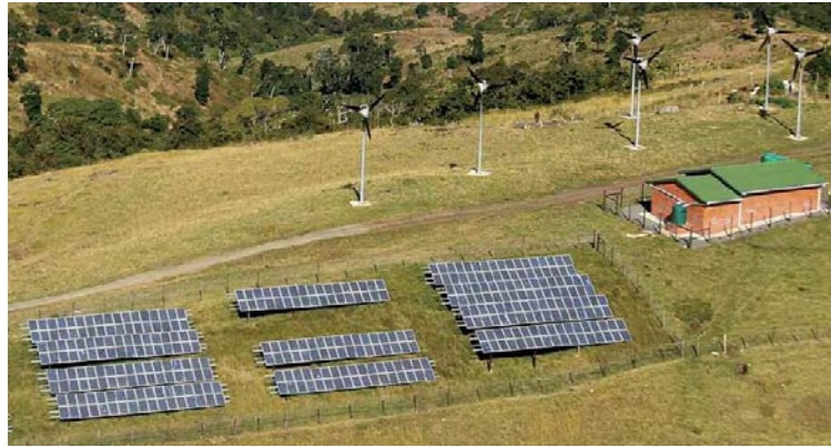
Figure 9. A mini-hybrid off-grid electricity system (PV and wind) at Lucingweni Village, South Africa (adapted from Rogers, 2009)
