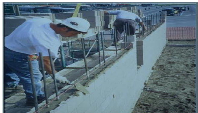
Figure 4. Reinforced Masonry Structure Construction in Canada [Bill McEwen]
