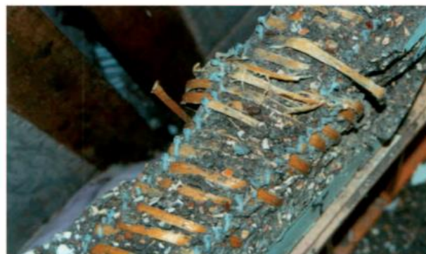
Figure 1. FRP spiral broke at failure.
