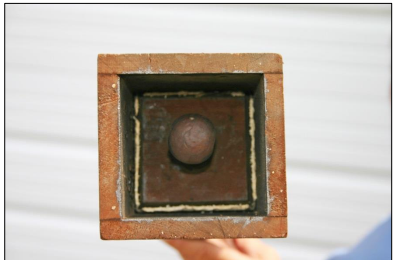
Figure 74 – The stop inside the wooden pipe.
