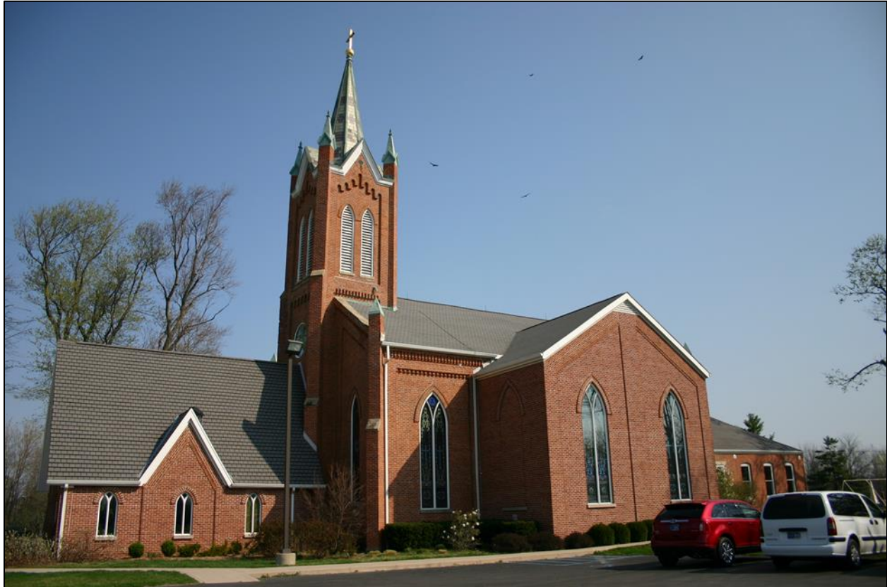
Figure 99 – Renovated St. Joseph Catholic Church, Hessen Cassel, IN (2001).
