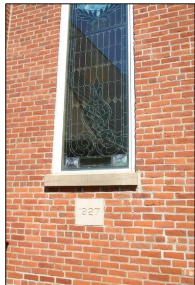
Figure 32 – St. Joseph’s Church, 1927 Stone Marker
