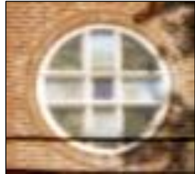
Figure 34 –Circular stained glass window replacement.
