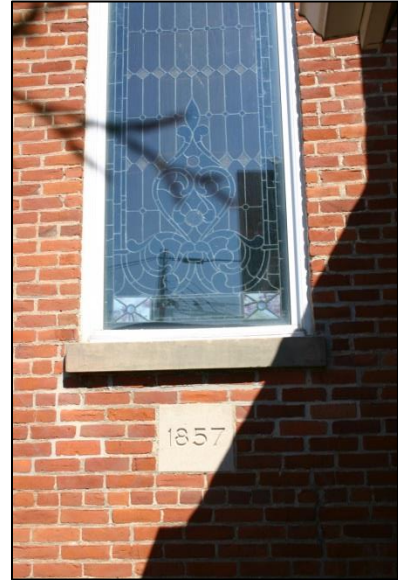
Figure 31 – St. Joseph’s Church, 1857 stone marker.
