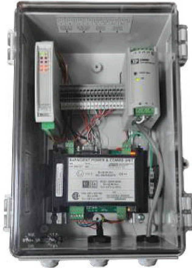
Inside of XIO showing I/O terminal block, power supply, and ExPAC
