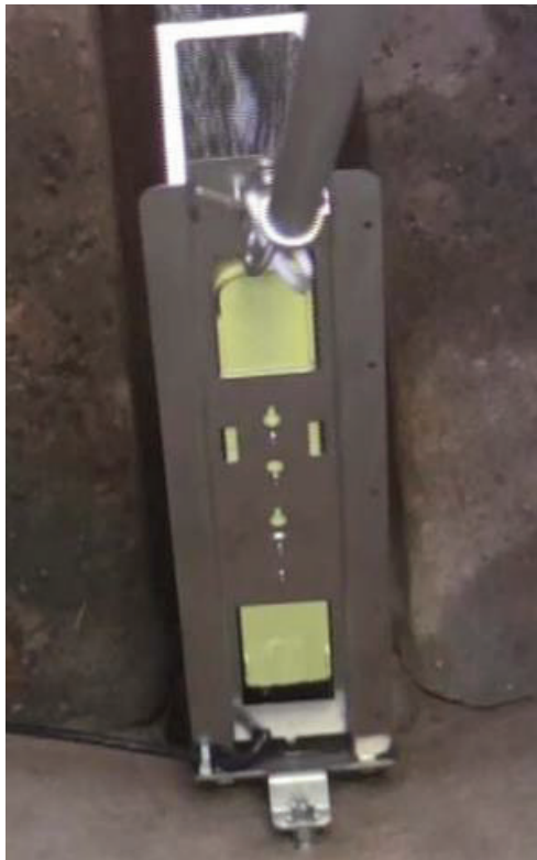
Turn the Hook Counter-Clockwise to Loosen and Raise Sensor Bracket
