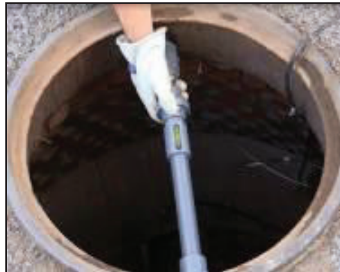
Positioning the Mounting Bar in the manhole frame
