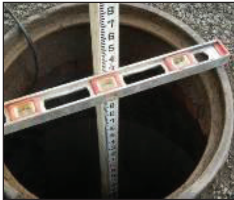
Placing Carpenter's level across open manhole frame
