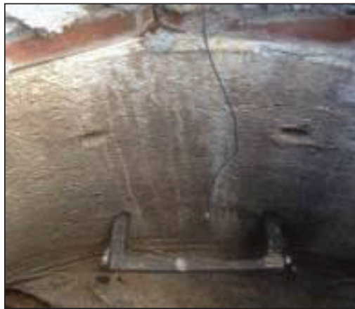
Passing Mounting Bar tether behind top rung
