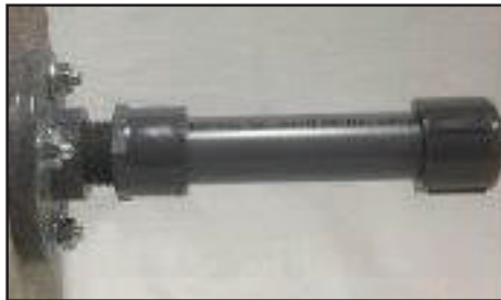
Screwing Wall Mount Bar into installed bracket
