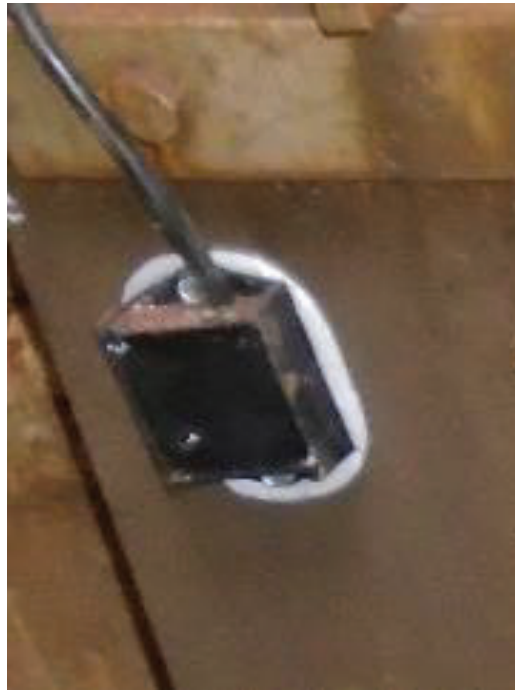
Inclinometer attached using Construction Adhesive
