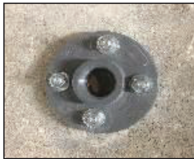
Securing bracket to the manhole wall
