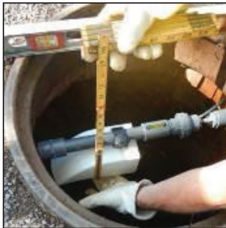
Placing Carpenter's Rule at base of sensor edge
