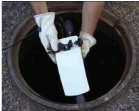
Unscrewing and opening shroud bracket
