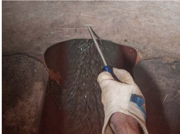
Mark Lower Tab Position for Mounting Bracket
