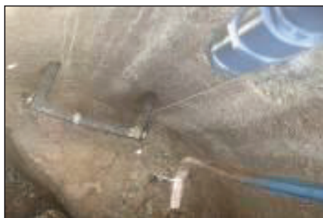
Using J-Hook to pull tether up from top rung
