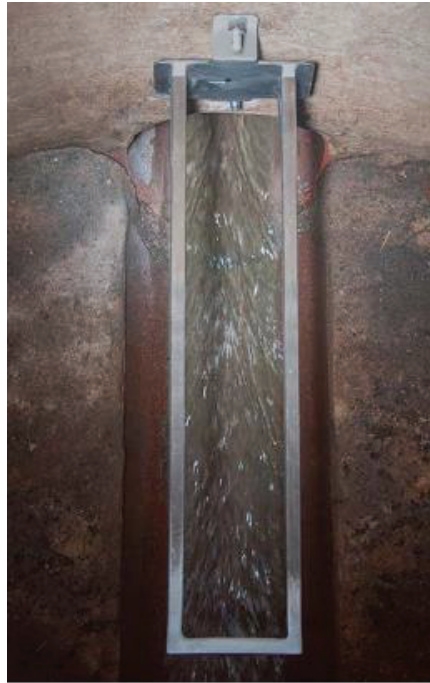
Installed ParaDepth/ParaFlow Wall Mount Bracket
