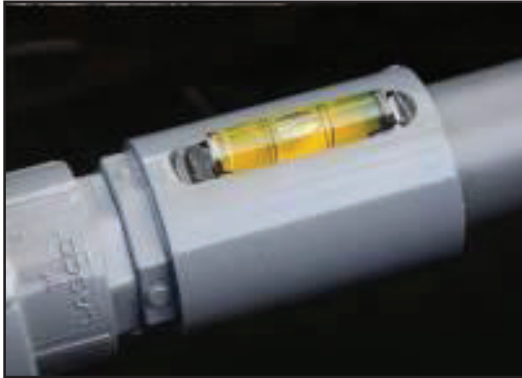
Ensuring Mounting Bar is level
