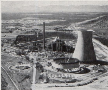
A view of Athlone Power Station under construction for Cape Town City Council
