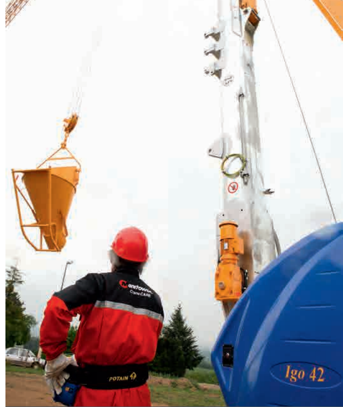
The crane operator is versatile thanks to the remote control.
