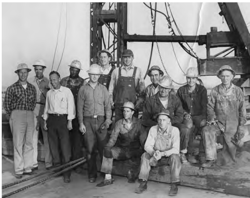
On one of his first jobs in the late 1950s, Oiler Robert Stefani, seated in the front row with gloves, works for Raymond Concrete Pile with his father, Crane Operator Pete Stefani, furthest in back. The project involved building storm drains in Rio Vista.
