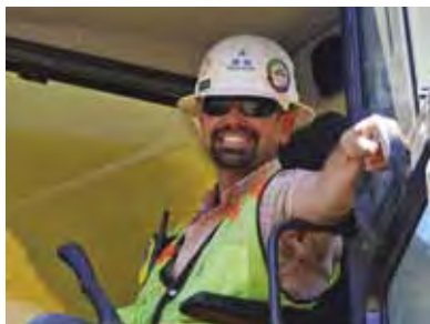
Jesse Johnson works on a levee project in Sutter County for Teichert Construction.
